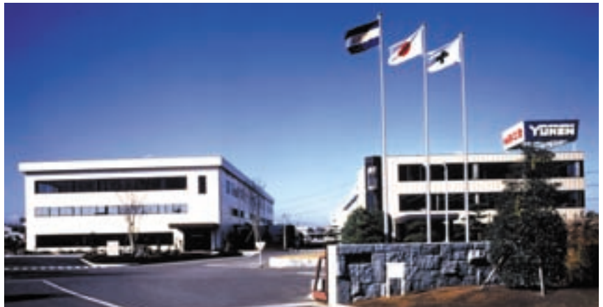
● Sagami Plant Front Gate
