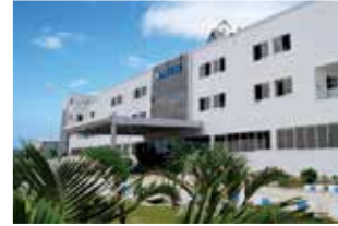
Rudrapur Plant (Green Building)
