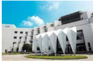
Tainan Plant (Diamond-rated Green Building)
