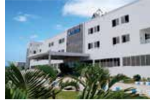
Rudrapur Plant (Green Building)
