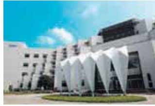
Tainan Plant (Diamond-rated Green Building)
