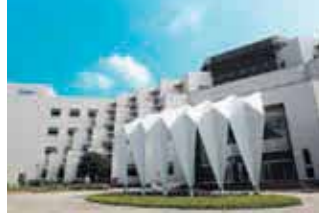
Tainan Plant (Diamond-rated Green Building)
