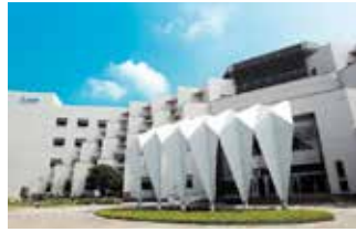
Tainan Plant (Diamond-rated Green Building)
